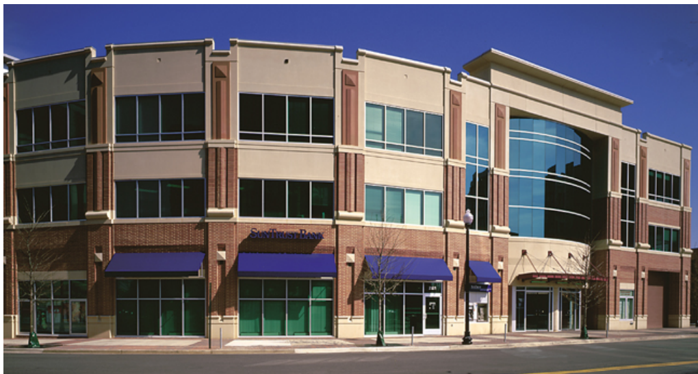
Courthouse Metro Plaza, Arlington, VA
